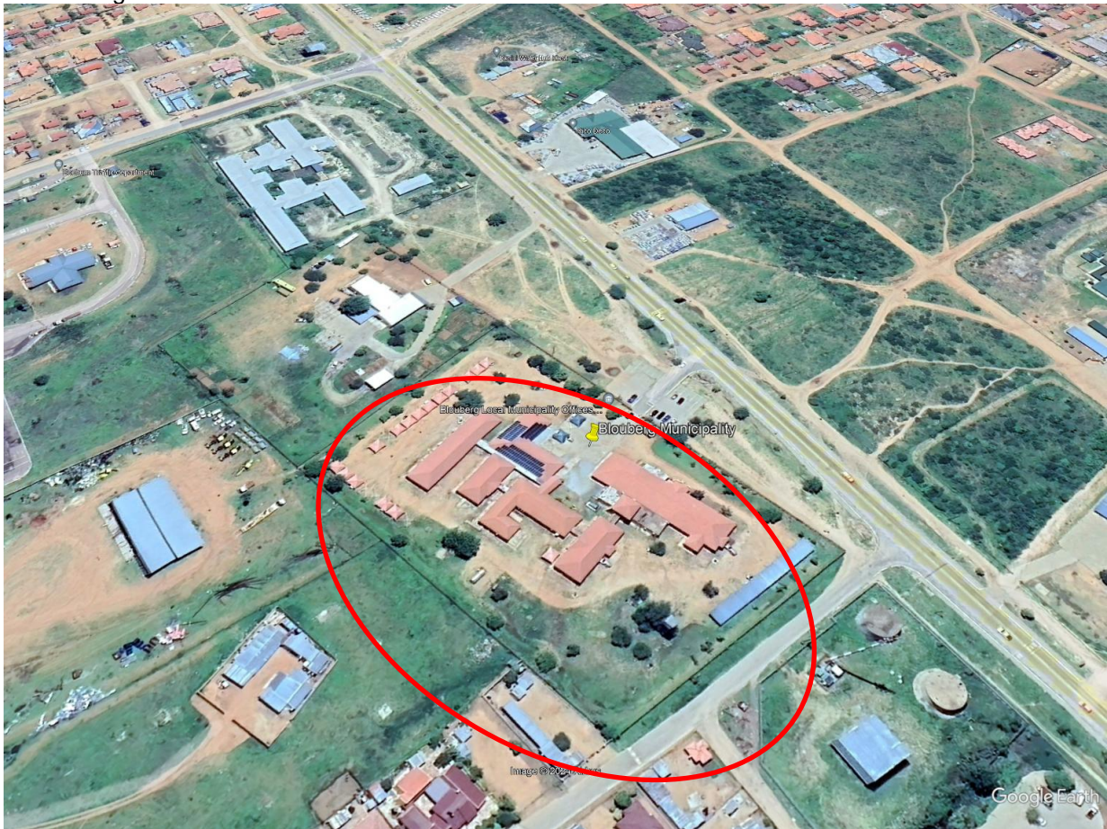
Figure 1 – Current Location of the Municipality
